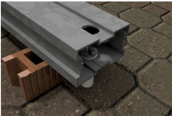
5. Batten screwed to the floor on a deck wedge.
