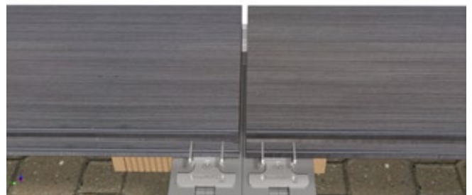
18. Installation of two battens between headers with a clip for each slat.
