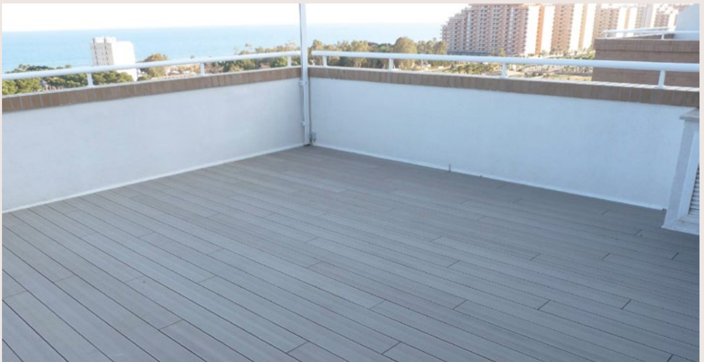
24. Assembled deck with invisible joint.
