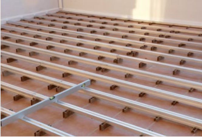
22. Batten installation for an invisible joint.
